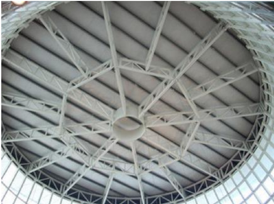
Figure 8: Building elements exposed
