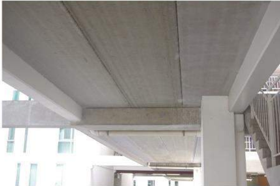
PRECAST CONCRETE COLUMNS,BEAMS AND FLOOR SLAB
