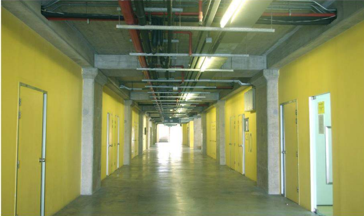
PRECAST CONCRETE COLUMNS,BEAMS AND FLOOR SLAB
