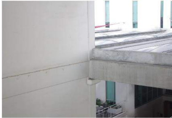
CONCRETE BEAM ON CONCRETE COLUMN
