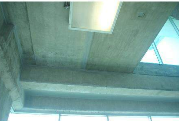
HOLLOWCORE FLOOR SLAB ON CONCRETE BEAM & COLUMN
