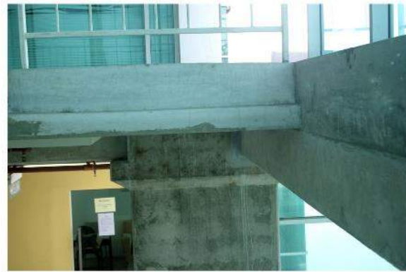
HOLLOWCORE FLOOR SLAB ON CONCRETE BEAM & COLUMN
