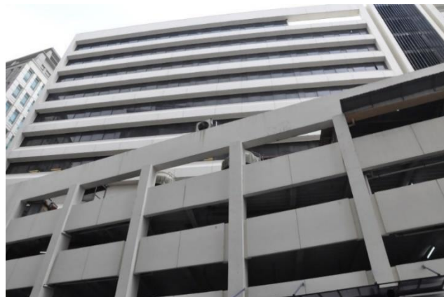
Figure 2.3.1.1.2: Façade of Wisma Antah
