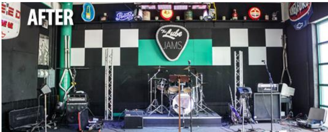
Figure 3.1.1.4: After treatment, concrete wall surface is covered with acoustical backdrop (Source: Soundproofing a Restaurant Case Study: Quaker Steak & Lube, 2014)
