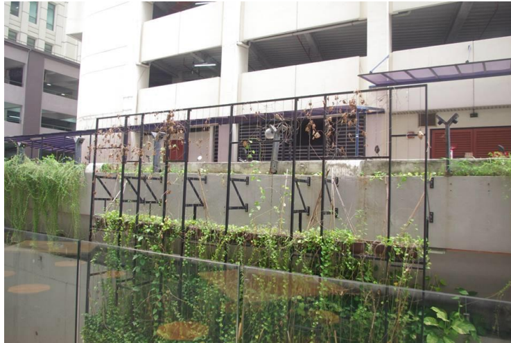
Figure 3.3.1.1.2: Outdoor dining area facing adjacent building's machine room
