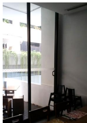
Figure 3.4.4.2.4: The glass panels located in Room 2
