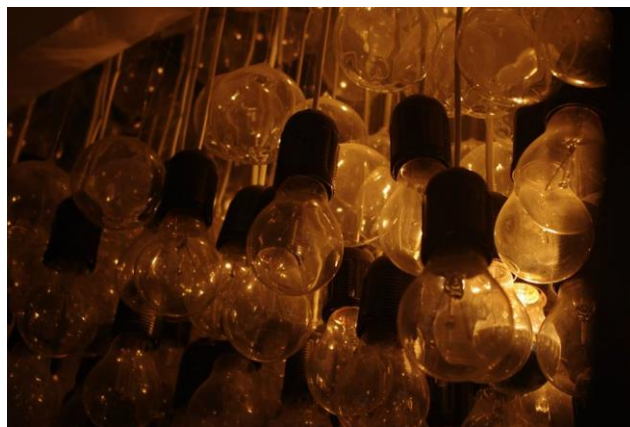
Figure 3.4.4.5.3: Large amount of decorative lights serve as sound absorber in the space
