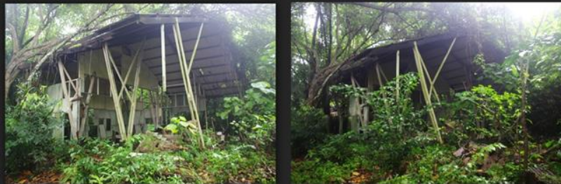
Former community hall for the residents
