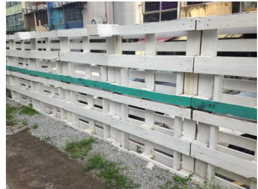
Figure 46 Wood pallets as the fencing gate. (Source: Mohammad Syarulnizam)
