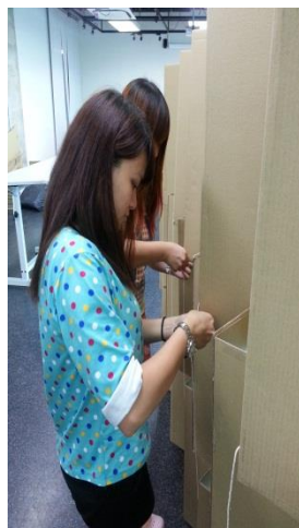
Figure 40 Attach string to strengthen the partition.
