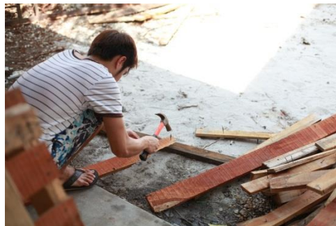
Figure 24 Removing all the nails on the wooden strip.
