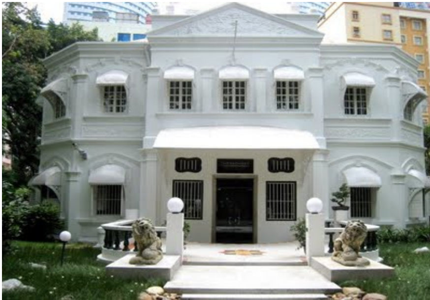
Figure 5.01 Front elevation of Loke Mansion (Source : Sreerema Banoo, 2009)
